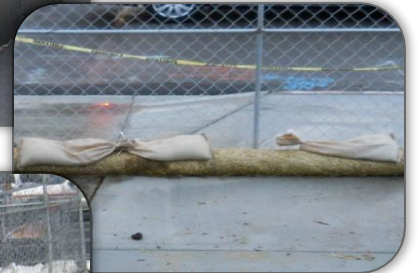
Fiber Rolls (trenched or secured)
