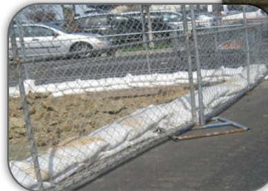
Gravel Bag Berm
